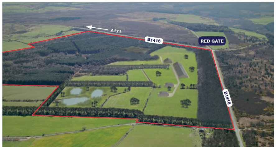
Aerial view looking south across site
